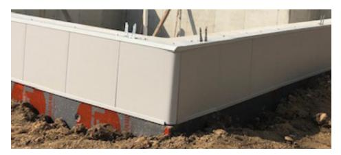
Corners and seams fit snug and look great. You can easily and quickly customize corners with a simple V-notch cut on the insulation.
